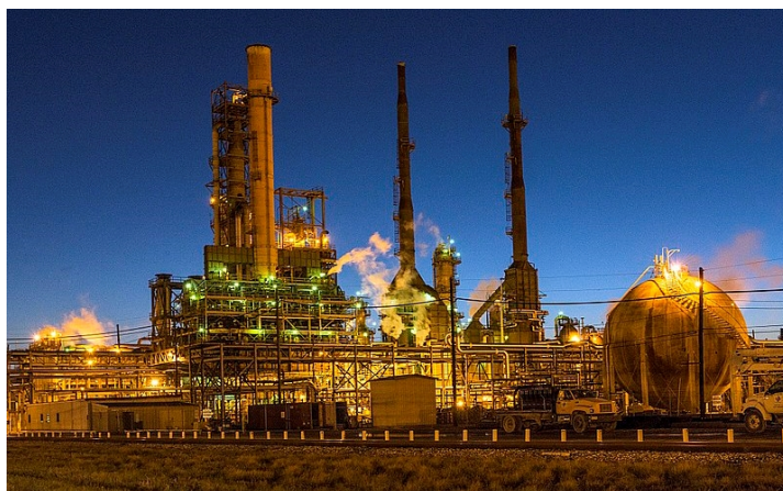
Figure 4 Valero Energy Corporation Refinery in Port Arthur, Texas 5
