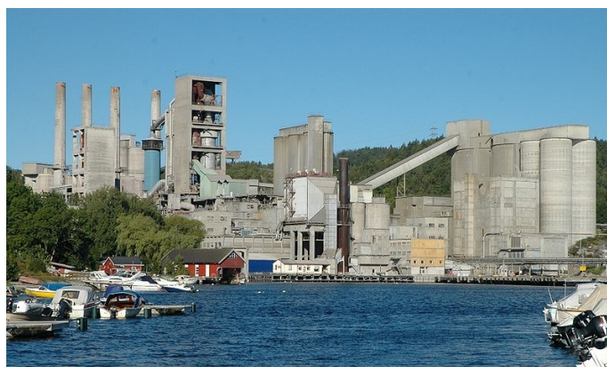
Figure 6 Norcem Brevik Cement plant 7
