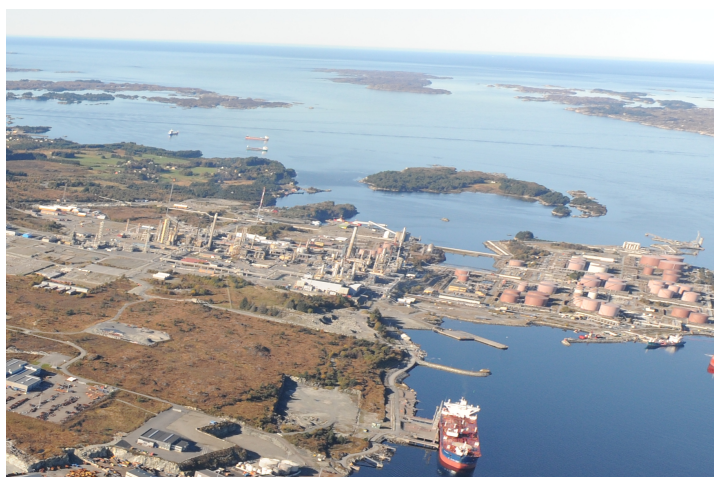
Figure 10 Air view of Mongstad area, where TCM is located 12
