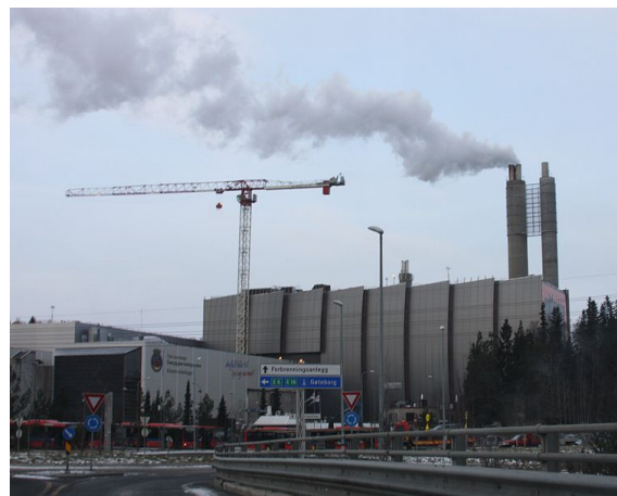
Figure 5 Klemetsrud Waste to Energy plant 6
