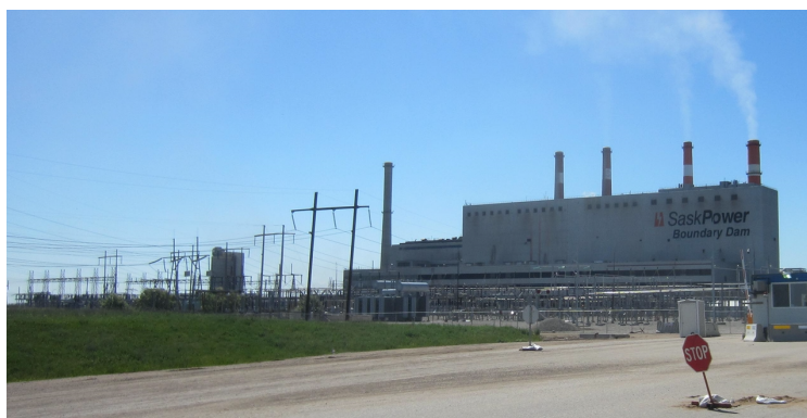
Figure 2 Boundary Dam Power Station Saskatchewan 3
