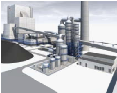
250 MWe Capture unit (post-combustion)
